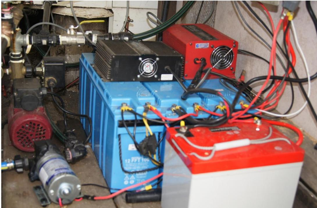
***The VK4NF Power & pumping station. 375ah battery capacity, that relates to about 200ah usable capacity. Thanks Wayne, the Batteries are working well. note the 12 volt water pump bottom left, and 240volt back up pump behind it.***
