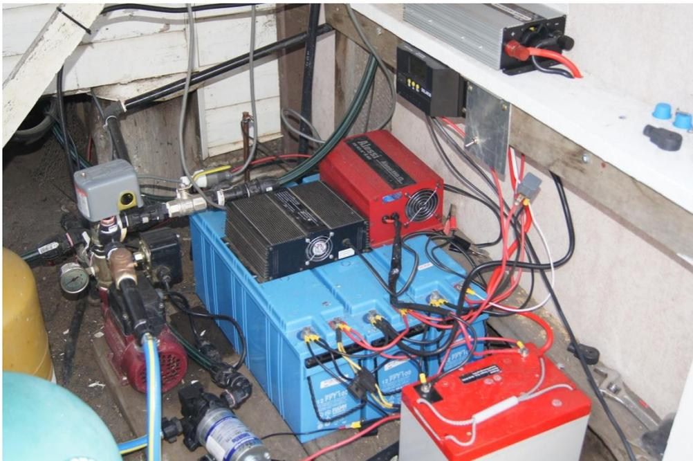
**Note the red inverter on the batteries, it generates noise for about a 4 mt radius of the station, The silver one sitting up on the shelf generates noise all around the property. they both work very well otherwise. Yes I know Albert, the red one is yours as is the charger beside it. they both work very well.**
